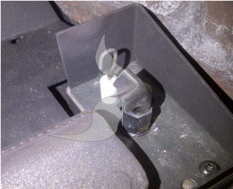
Figure 21. Correct Burner & Pilot Shield Placement
