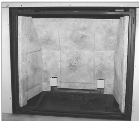
Figure 14: Right Firebox Liner Panel in Place.
