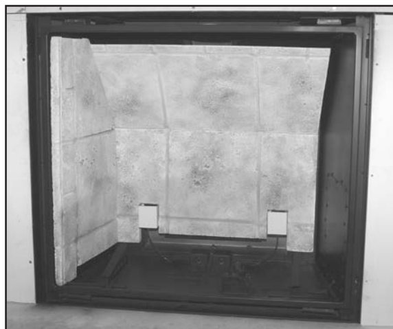
Figure 13: Top Firebox Liner Panel in Place.
