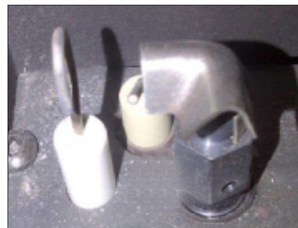
Figure 28 Proper Pilot Position
