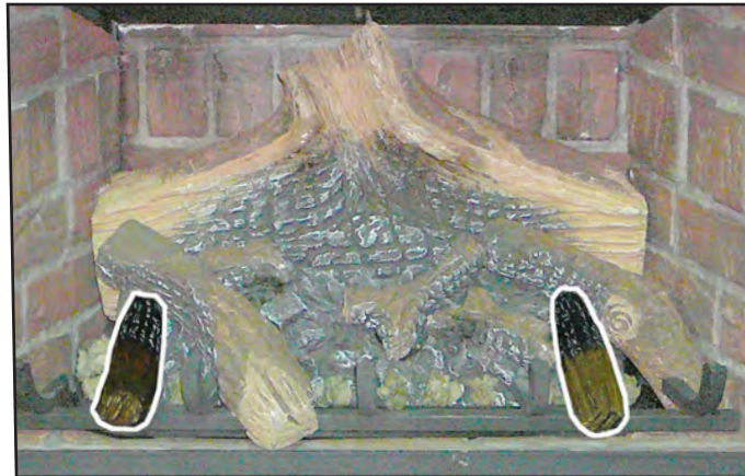
Figure 54. Sixth Stage Log Set Installation.
