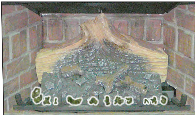
Figure 52. Fourth Stage Log Set Installation.
