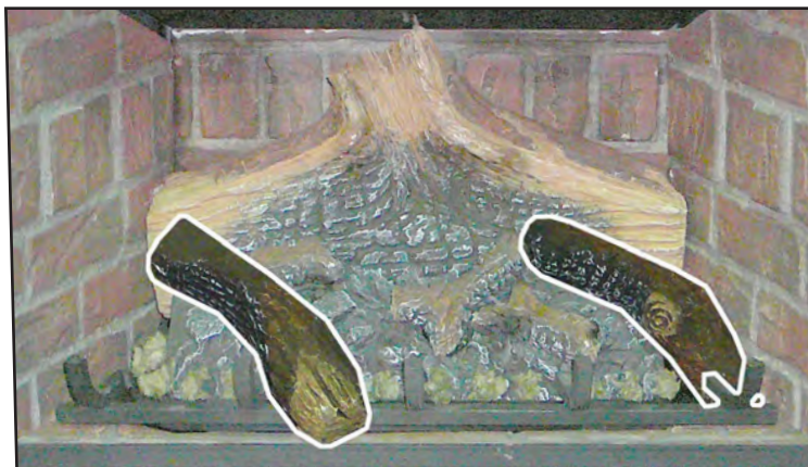
Figure 53. Fifth Stage Log Set Installation.
