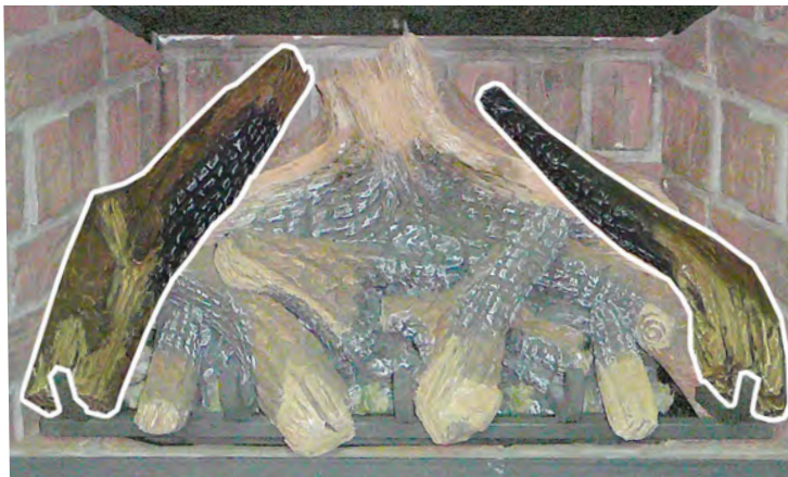
Figure 56. Eighth Stage Log Set Installation.
