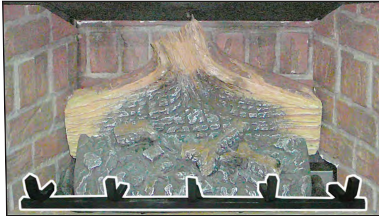
Figure 51. Third Stage Log Set Installation.
