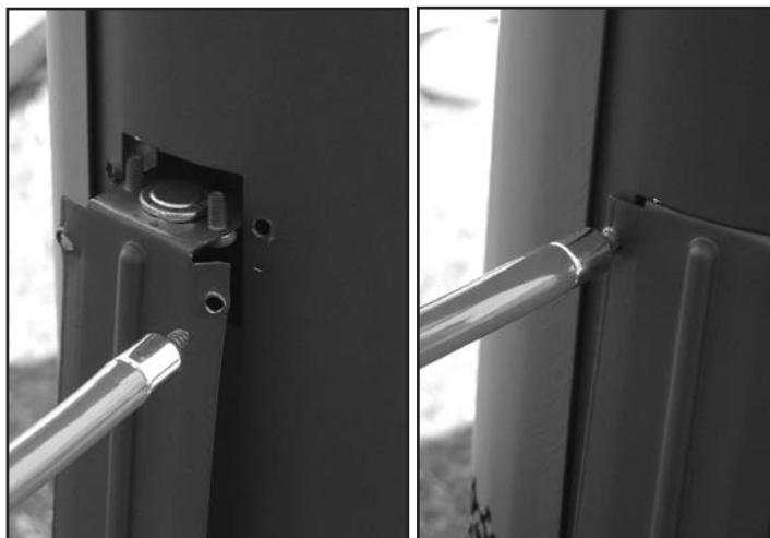
Figure 40: Spill switch installation.
