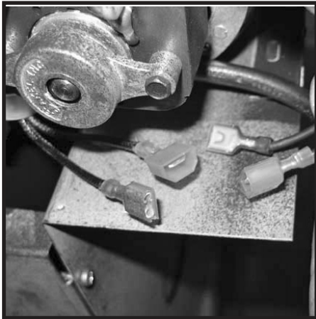
Figure 13: Disconnecting fan wires.
