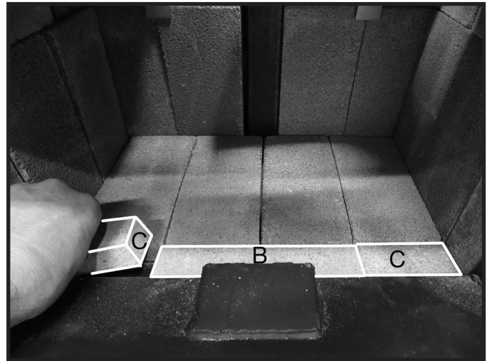
Figure 19: Narrow front bricks in place.
