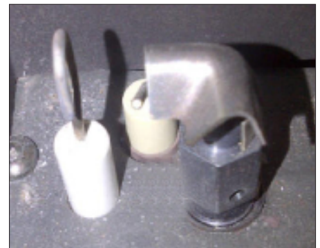
Figure 28: Correct Pilot Position
