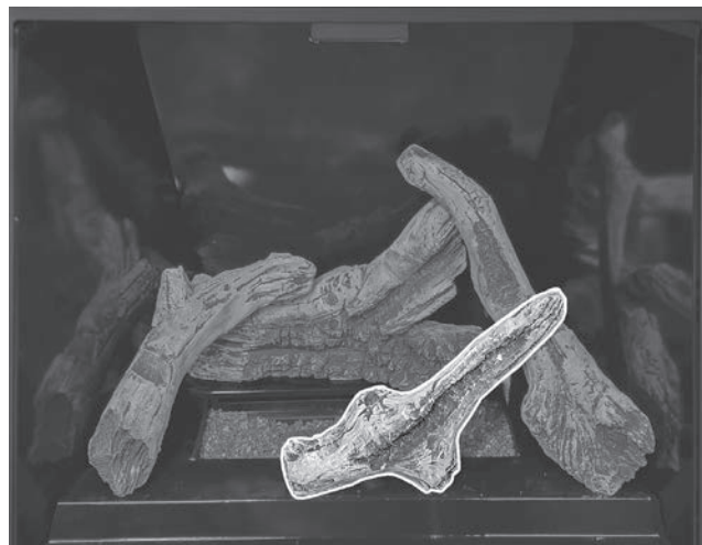
Figure 81: Log Set Installation - Step 9
